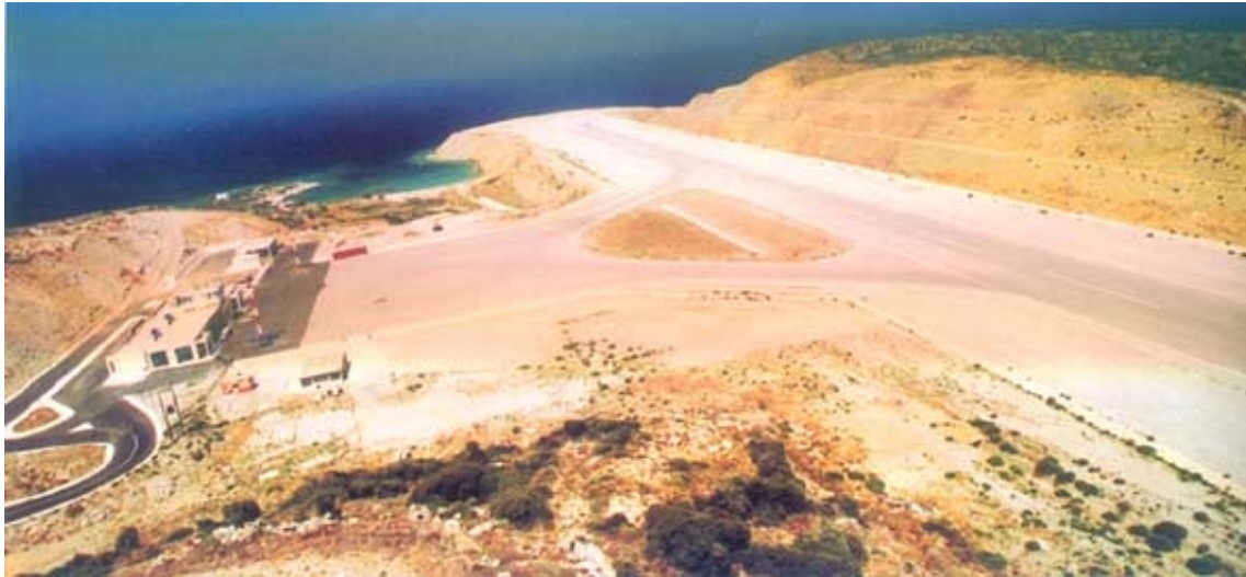
FIG. 1. The runway of the Ikaria airport is oriented NNE-SSW and terminated on an embankment area near the coast. At this area the runway was planned to be extended. (photo: Air Traffic Safety Electronic Engineers Association of Hellenic Civil Aviation Authority: http://www.hcaa-eleng.gr/ikaria.htm )
